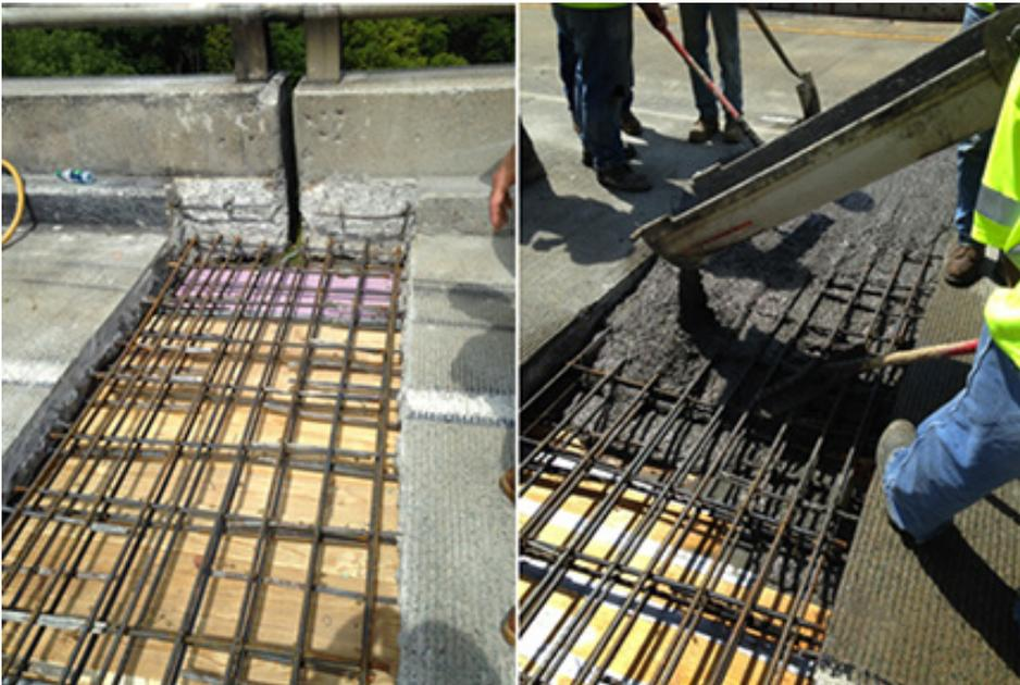
Fig. 7 and 8. Remove Concrete in Deck for 2' on Either Side of Joint; Form Between Girders; Place Bondbreaker (foam) over Girders; Place Reinforcement; Cast Concrete
