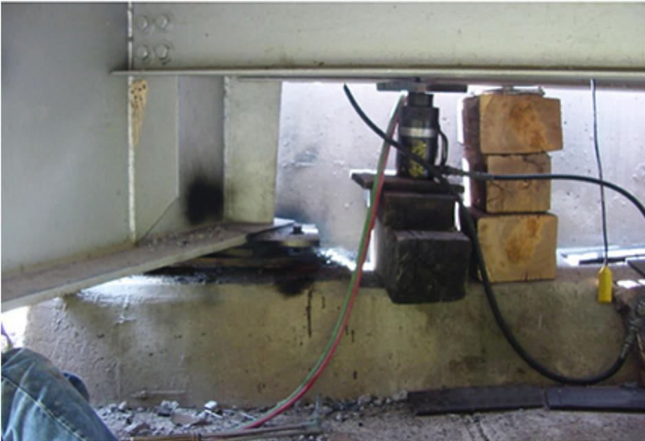
Fig. 6. Step 1 - Jacking Beam Ends to Free Bearings
