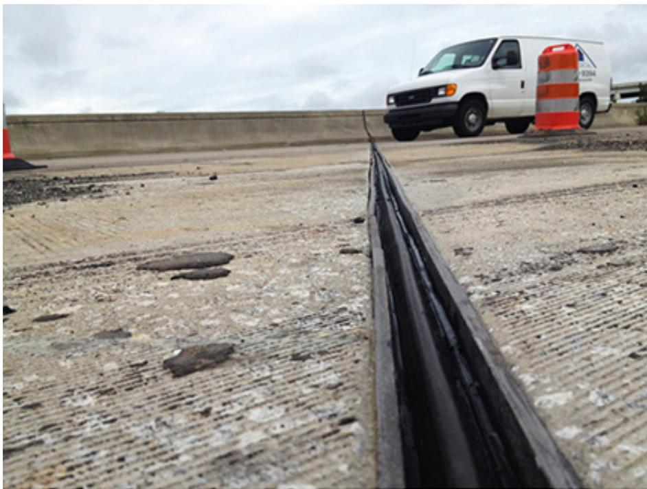
Fig. 1. A close up of a preformed silicone bridge joint system.
