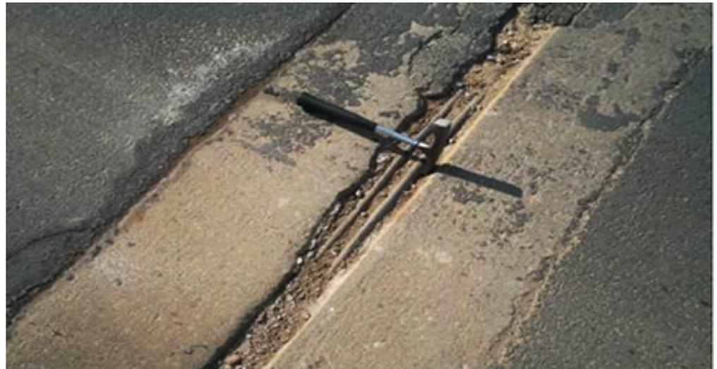
Fig. 1. Typical Bridge Deck Expansion Joint.
