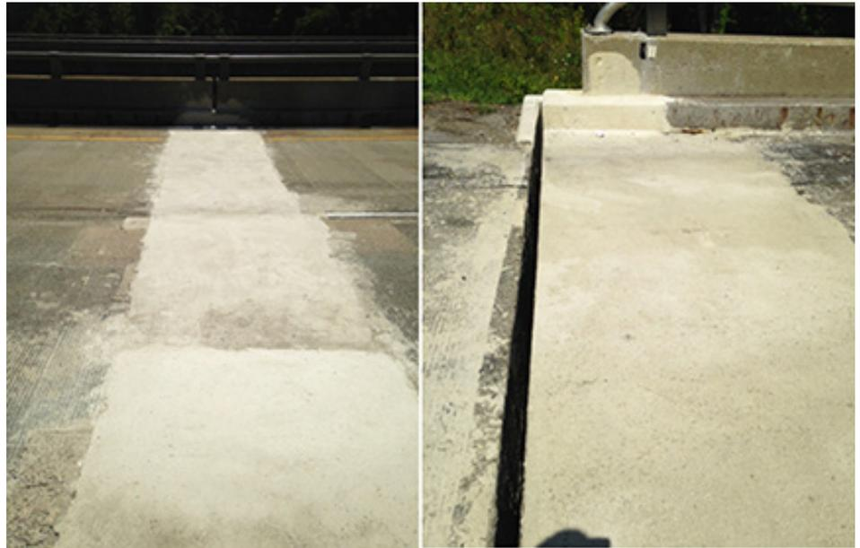
Fig. 9 and 10. Joints Eliminated Over Pier and at Abutment
