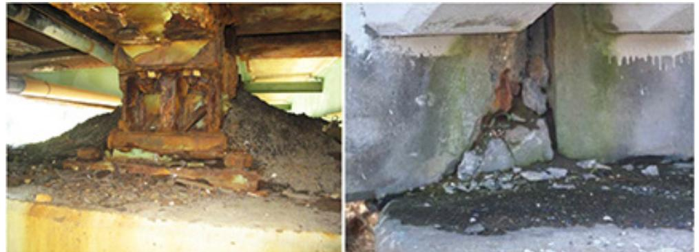
Fig. 2 and 3. Corrosion, Deterioration and Sediment Buildup Under Leaking Joints
