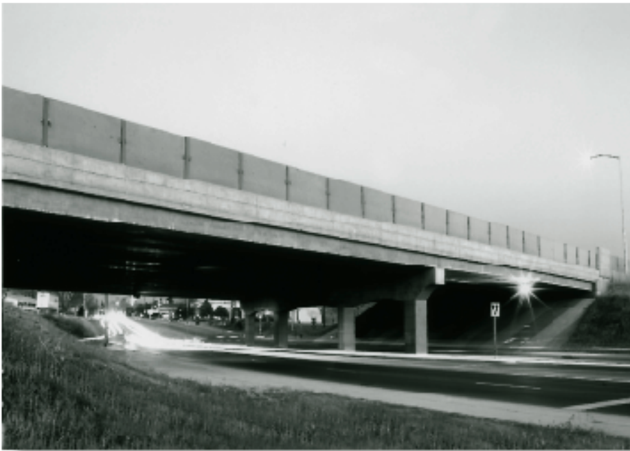
HPC resulted in a longer span-to-depth ratio and improved sight distance.
