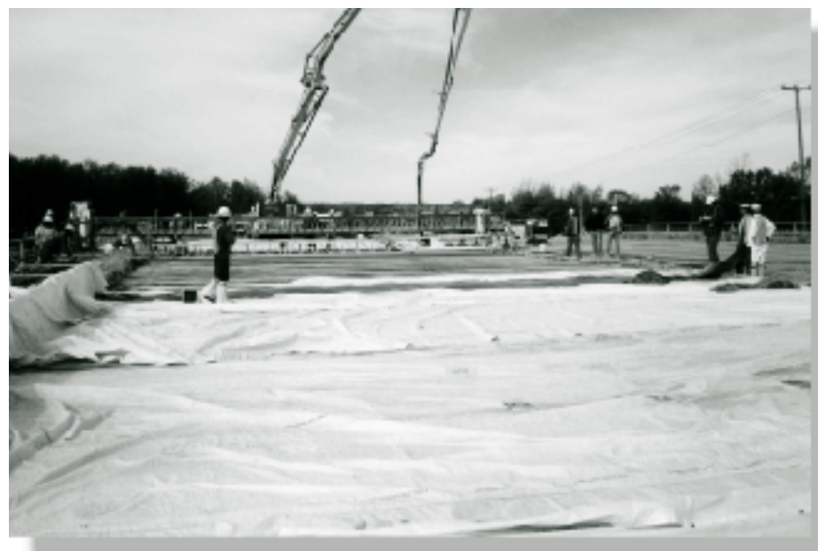
Construction of a low permeability bridge deck in Virginia.
