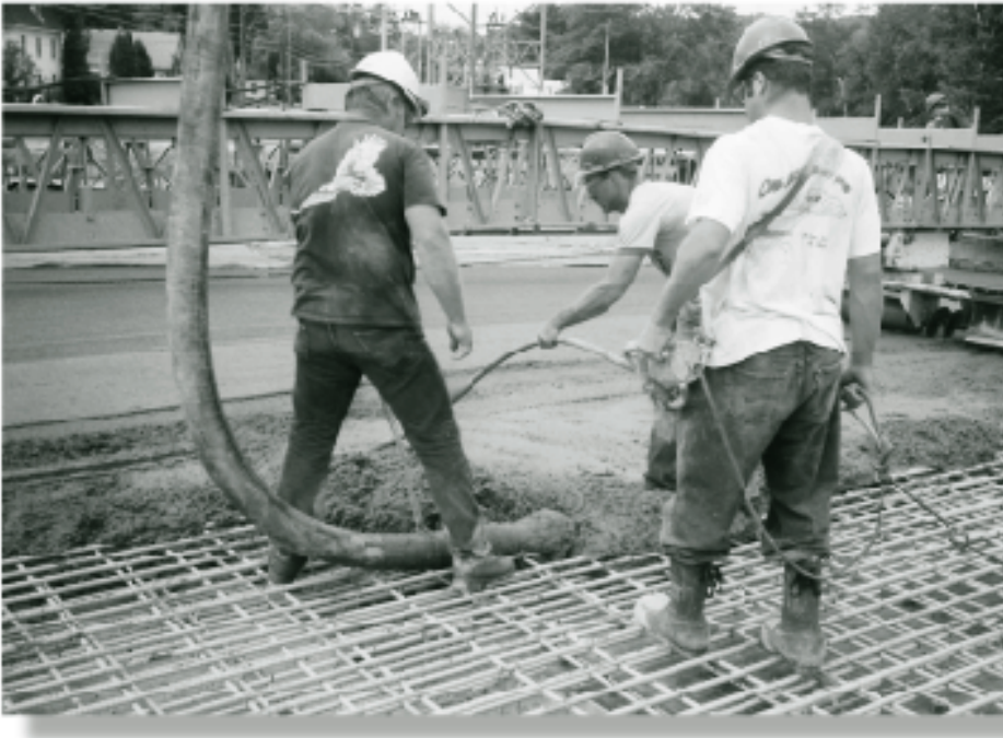
Placing concrete on New Hampshire's HPC bridge deck.
