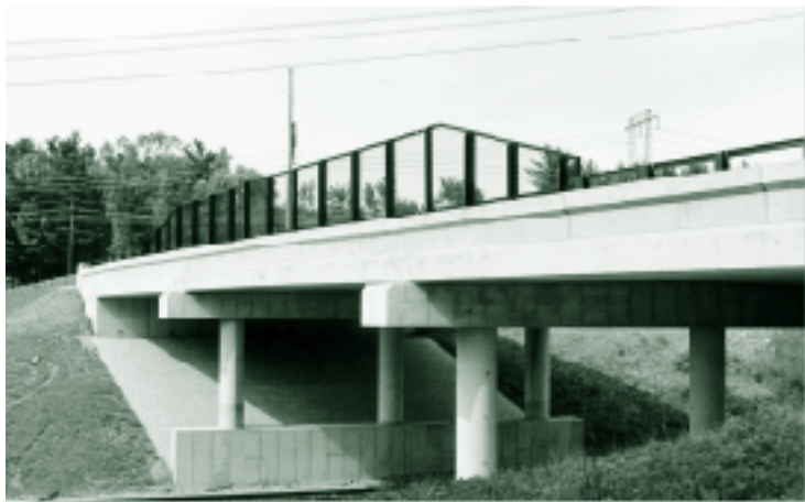
HPC was used to enhance durability of the cast-in-place superstructure components.
