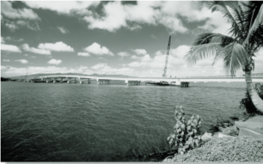
HPC was used on the Admiral Clarey Bridge to meet the Navy's requirement for a durable structure.
