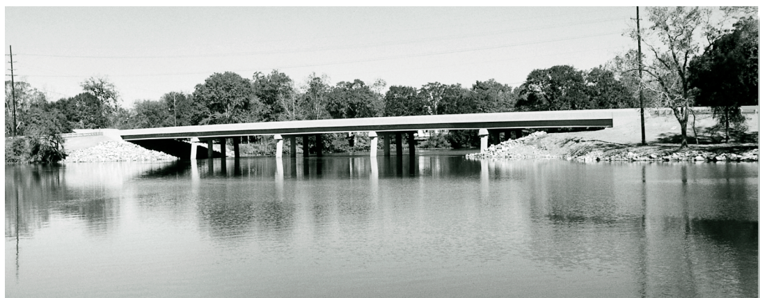
HPC was used in substructure and superstructure for strength and durability.
