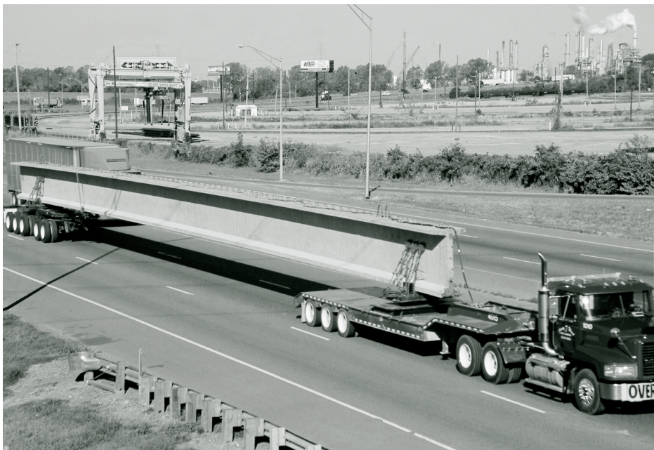
Hauling a 156-ft (47.5-m) long HPC girder to the jobsite.
