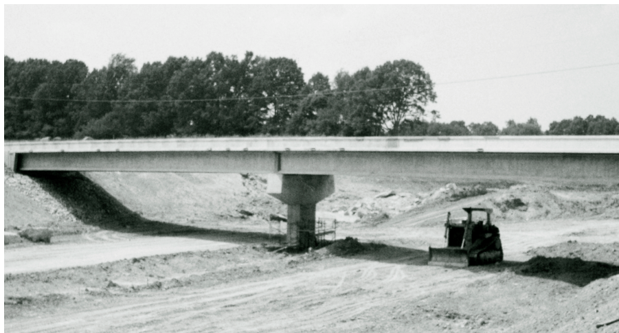
HPC allowed the use of wider beam spacings and resulted in more economical bridges.
