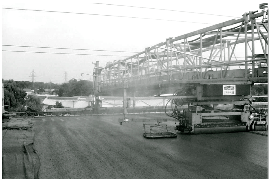
Fogging equipment attached to the finishing equipment.
