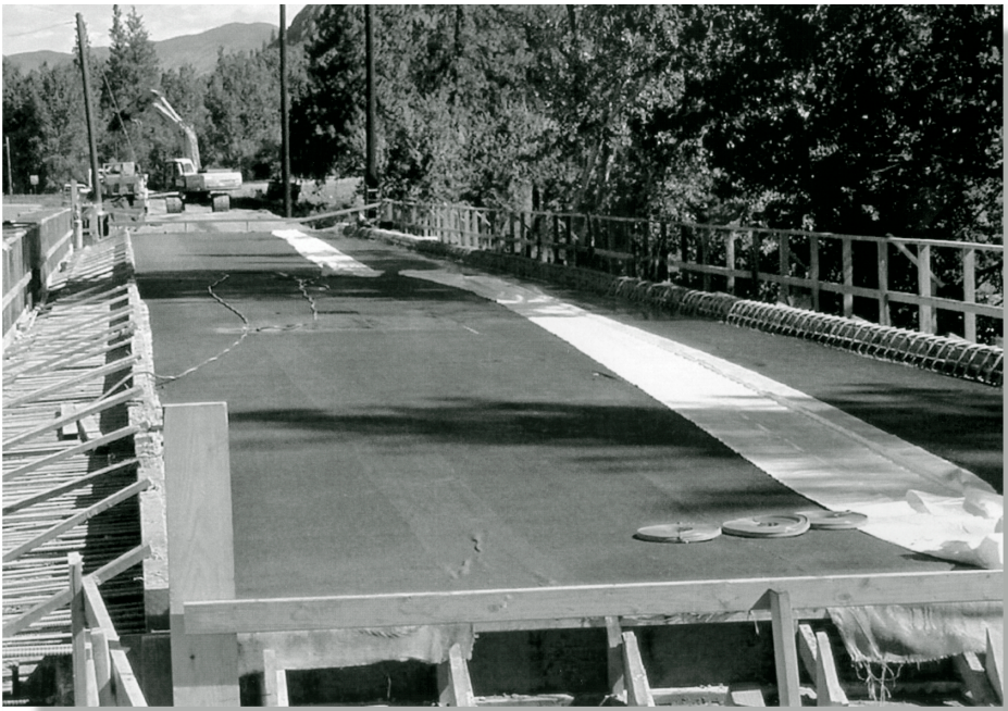
Continuous wet curing is required for 14 days.
