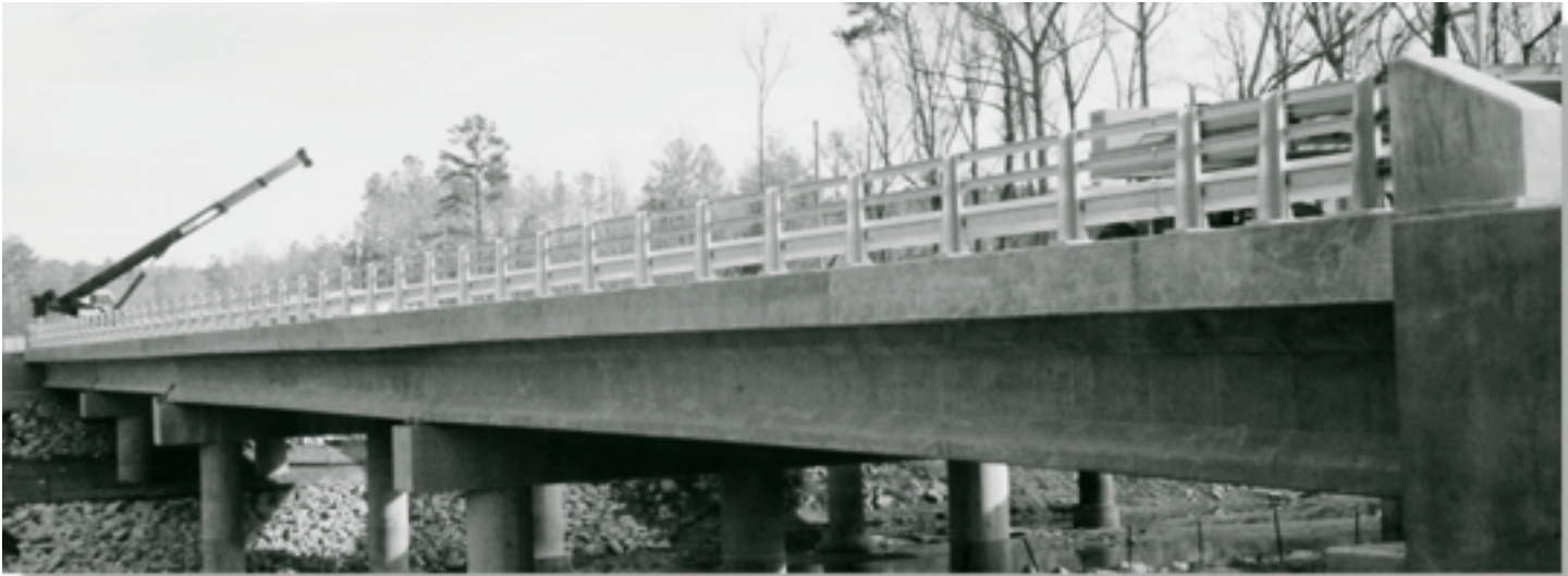
HPC was used in the girders and deck of the northbound and southbound bridges.
