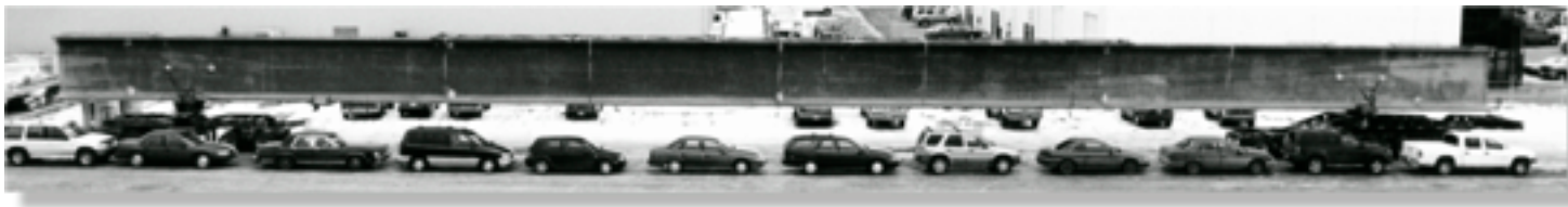
Pretensioning, post-tensioning, and high-strength concrete were used to achieve a record length. (Photo courtesy of Con-Force.)
