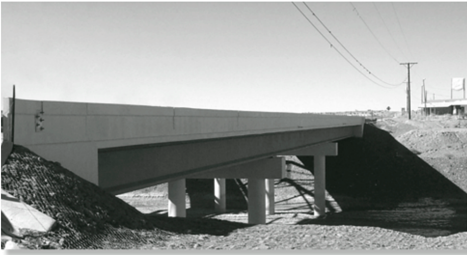
The viability of using HPC in New Mexico was established with construction of the Rio Puerco Bridge.
