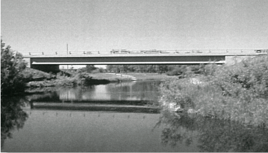
Precast, prestressed concrete was selected for its shorter delivery and erection time.
