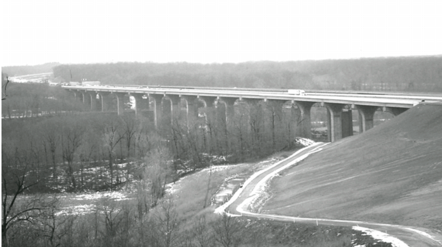
HPC, epoxy-coated reinforcement, and a silane sealer were used to provide a durable deck.
