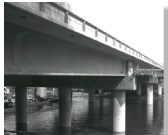
HPC spliced bulb-tee girders were used to satisfy the project constraints.
