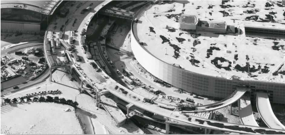
Preblended silica fume cement and slag cement were used to obtain a 50-year service life.
