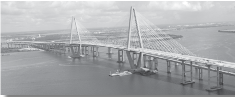
HPC was used in many components of the Cooper River Bridge (Photo courtesy of SCDOT/Rob Thompson)
