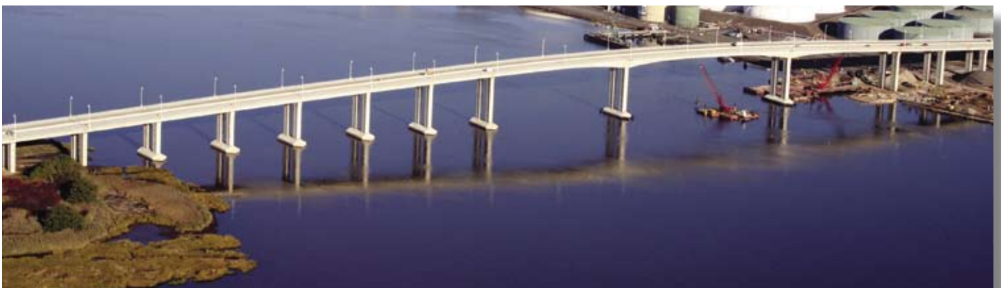
HPC was used in the foundations, piers, and superstructure of the new Victory Bridge. Photo ©FIGG.
