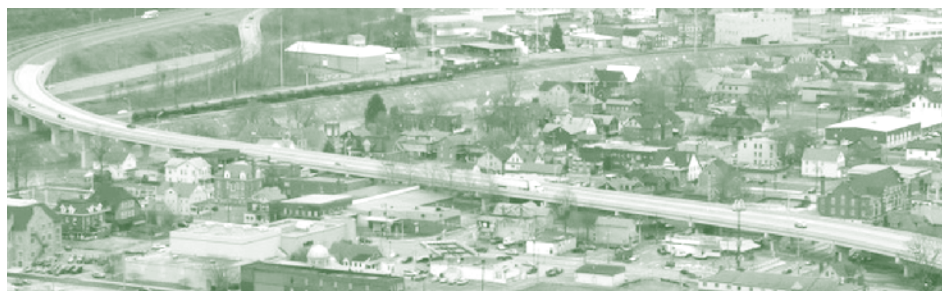
Bridge deck cracking on the Kernville Viaduct was reduced by 62 percent.
