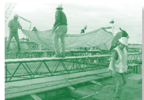
Two layers of burlap must be placed within 15 minutes of finishing.
