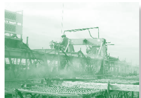
Fogging equipment is mounted on the finishing equipment.
