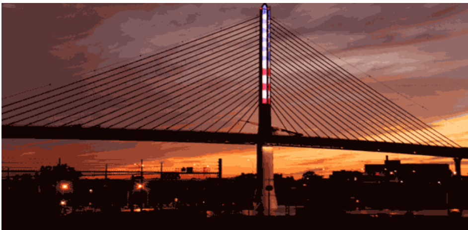
The pylon of the Veteran's Glass City Skyway used 10,000 psi (69 MPa) mass concrete.
