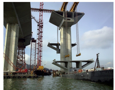
Erection of precast concrete segments from a barge.
