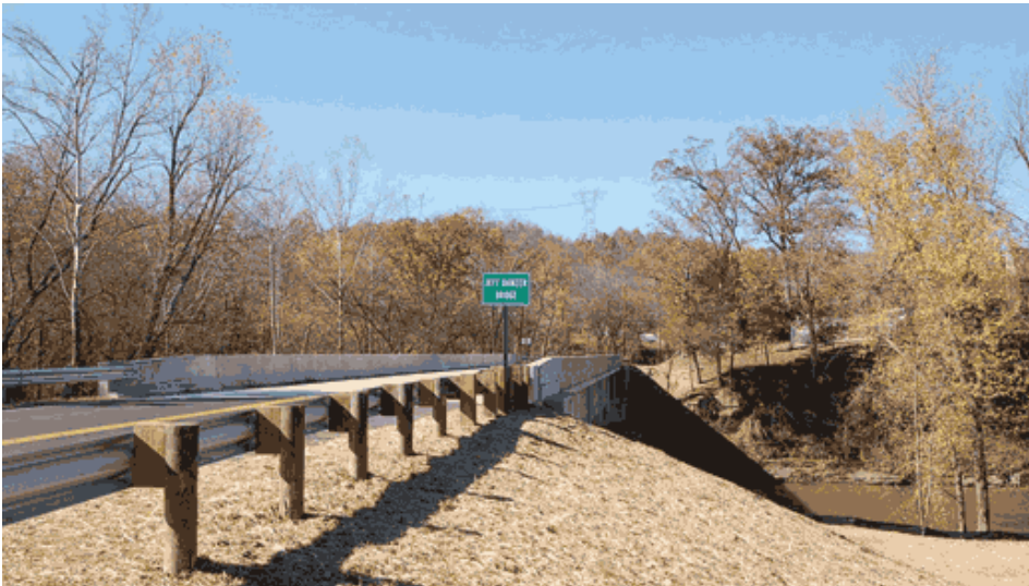
Sand-lightweight concrete was used to reduce the shipping and handling weight of the precast, prestressed concrete beams.
