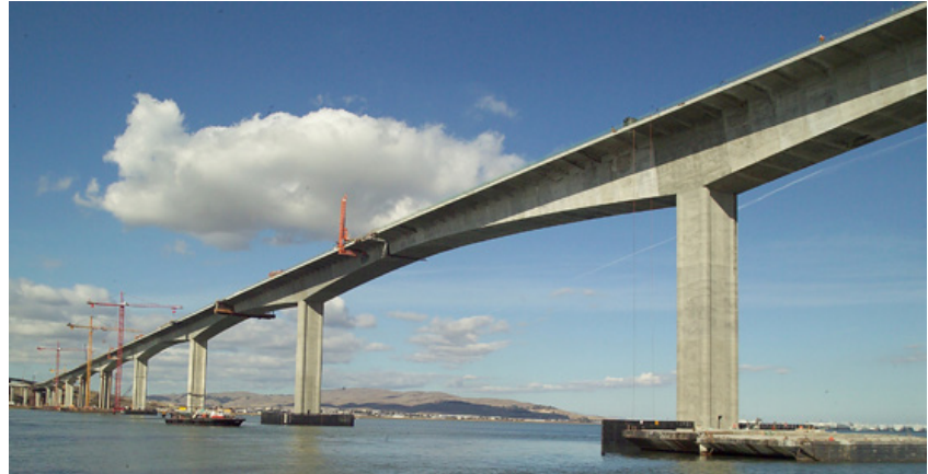
Lightweight high performance concrete was used for the cast-in-place superstructure segments.
