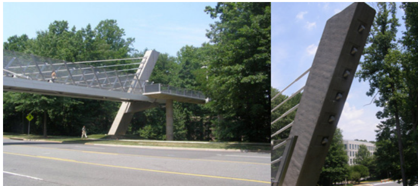
SCC was used in the inclined pylons of the cable-supported pedestrian bridge, VA. Photos: Virginia Department of Transportation.
