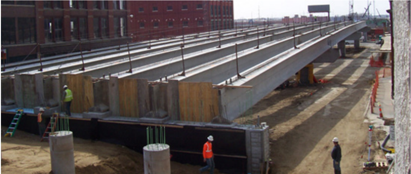
Self-consolidating concrete with a compressive strength of 12,000 psi (83 MPa) was used in the beams of the Harris Overpass, Lincoln, NE.
