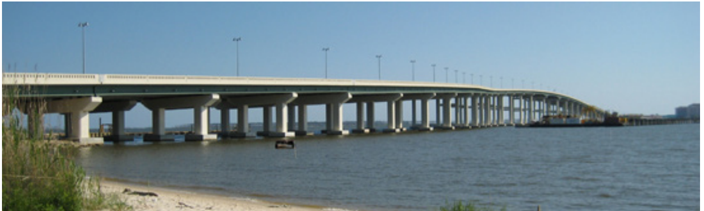
Self-consolidating concrete was used in the precast, prestressed concrete beams of the new Biloxi Bay Bridge.
