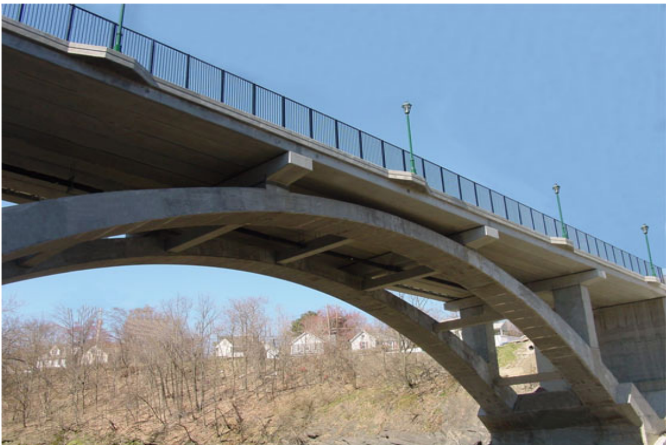
Route 52 bridge over the Wallkill River
