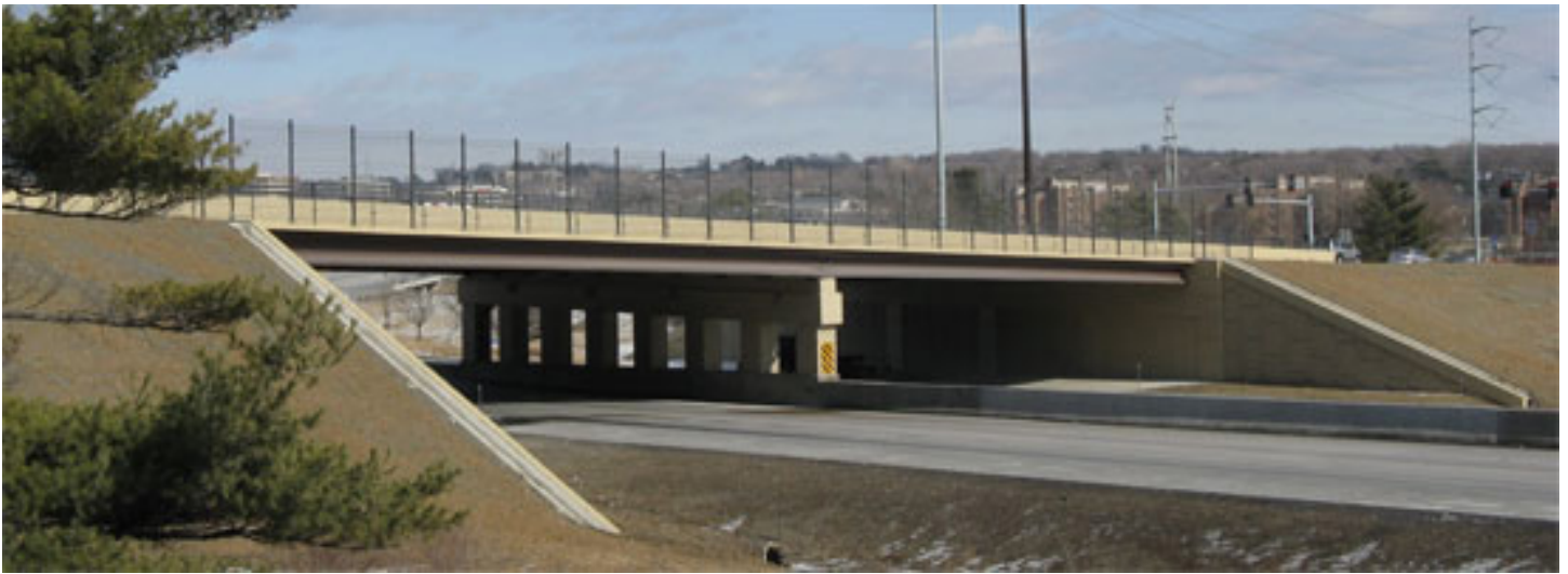
High strength concrete and 0.7-in. (17.8-mm) diameter strands were used in the precast, prestressed concrete beams.
