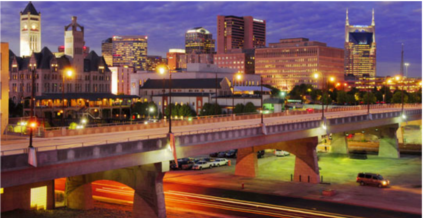
High strength concrete was used in the box beams to achieve a span-to-depth ratio of 29.
