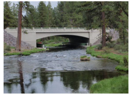
Replacement Collier's Promenade Bridge
