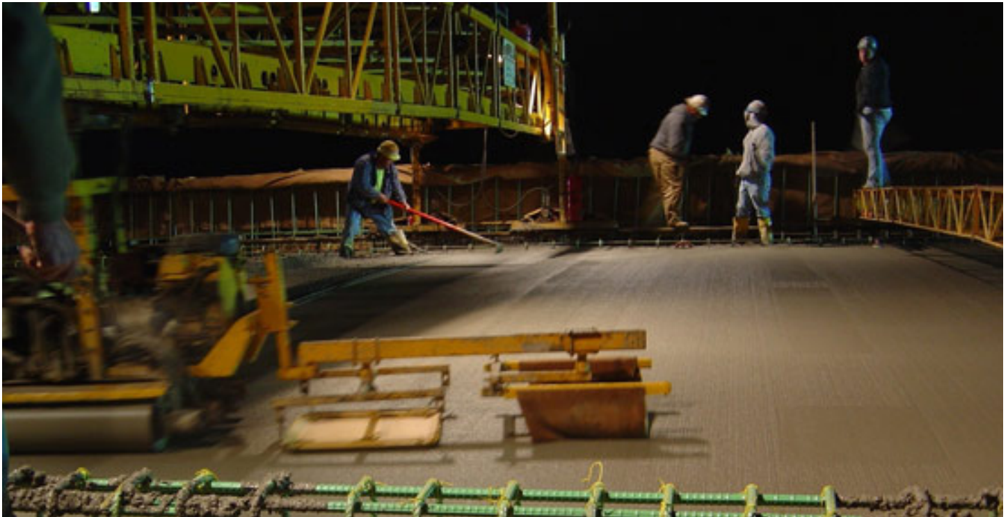
High strength concrete was used in the box beams to achieve a span-to-depth ratio of 29.
