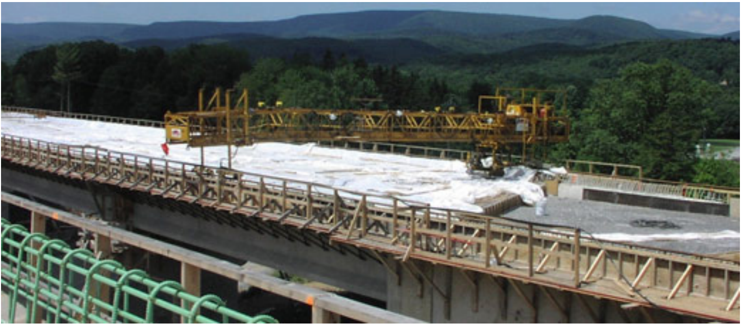
Curing of concrete bridge decks requires saturated burlap for 7 days.
