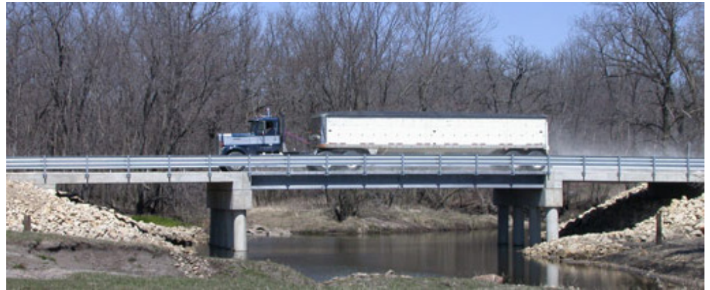
The center span of this bridge in Buchanan County utilized UHPC.
