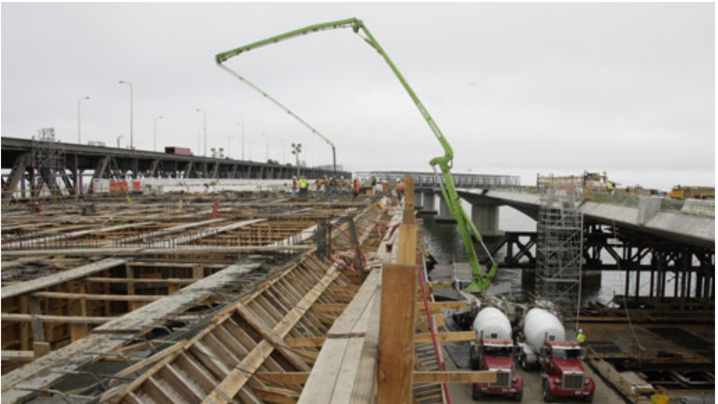
The concrete on the San Francisco-Oakland Bay Bridge made extensive use of fly ash. Photo: California Department of Transportation
