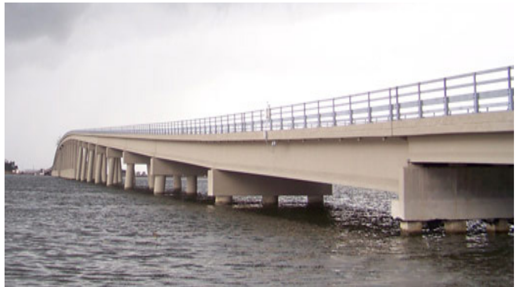
HPC was used in the girders of two spans of the Rigolets Pass Bridge.
