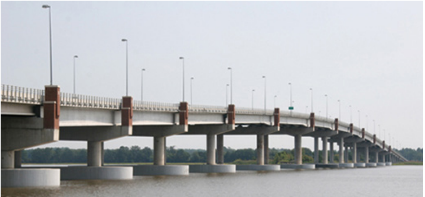
High strength lightweight concrete was specified for the Route 33 Bridge over the Mattaponi River, VA.
