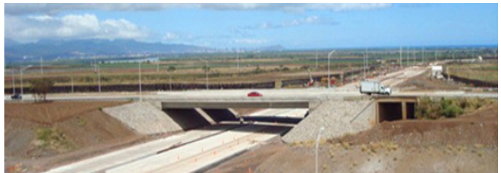
HPC was used in the spliced beams and deck.
