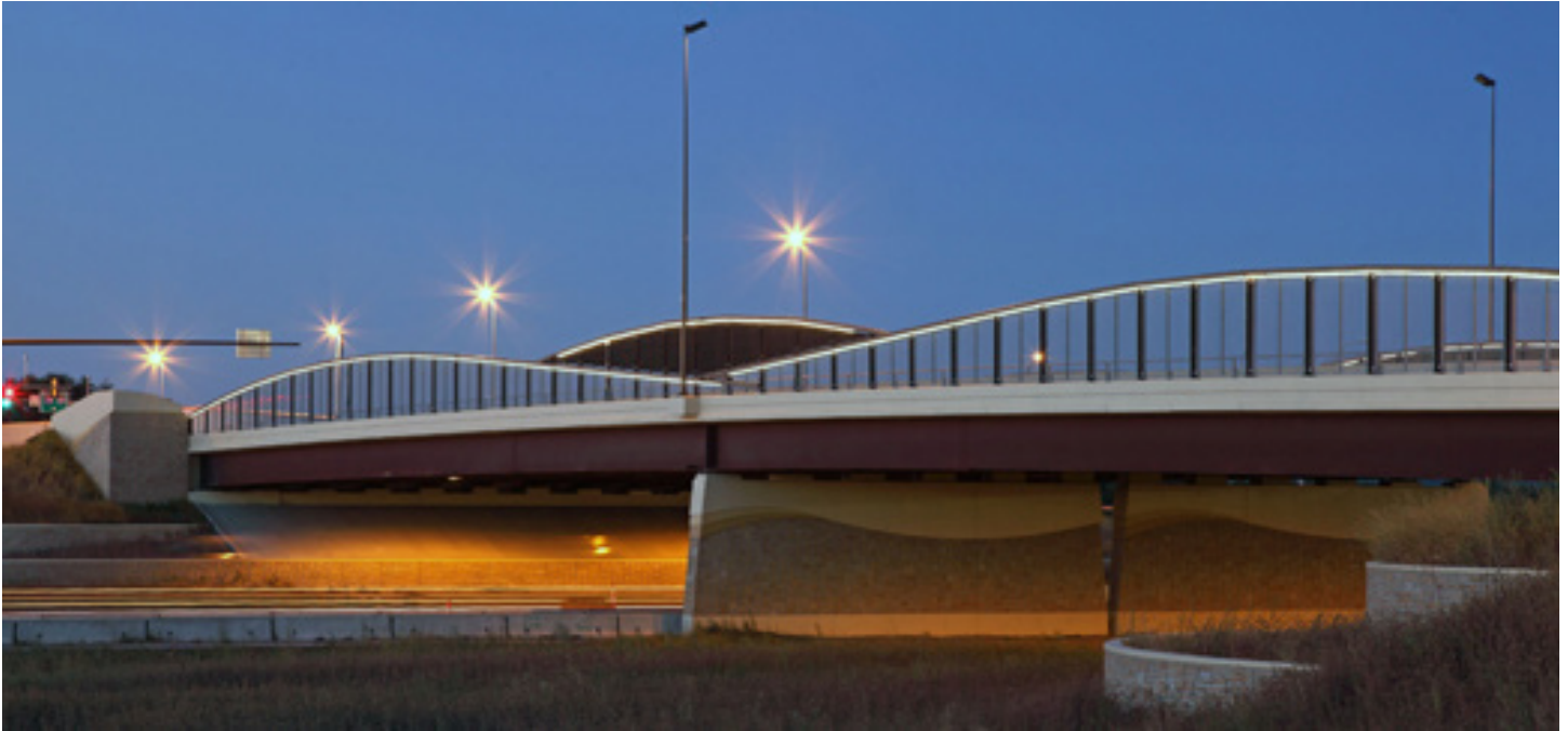
24th Street Bridge, Council Bluffs, IA. Photo: Keith Philpott
