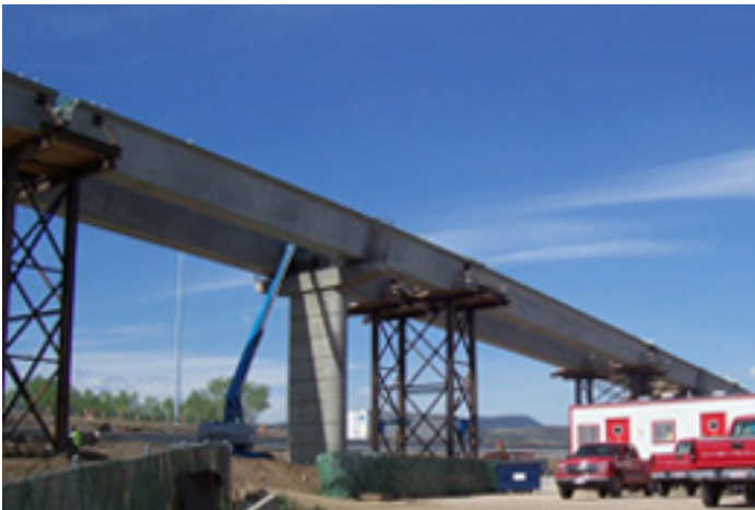
High strength, flowable concrete was used in the curved and straight girders.
