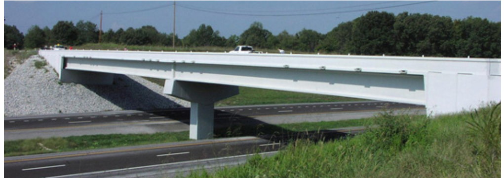
HPC was used in the superstructure of the Hickman Road Bridge, TN.
