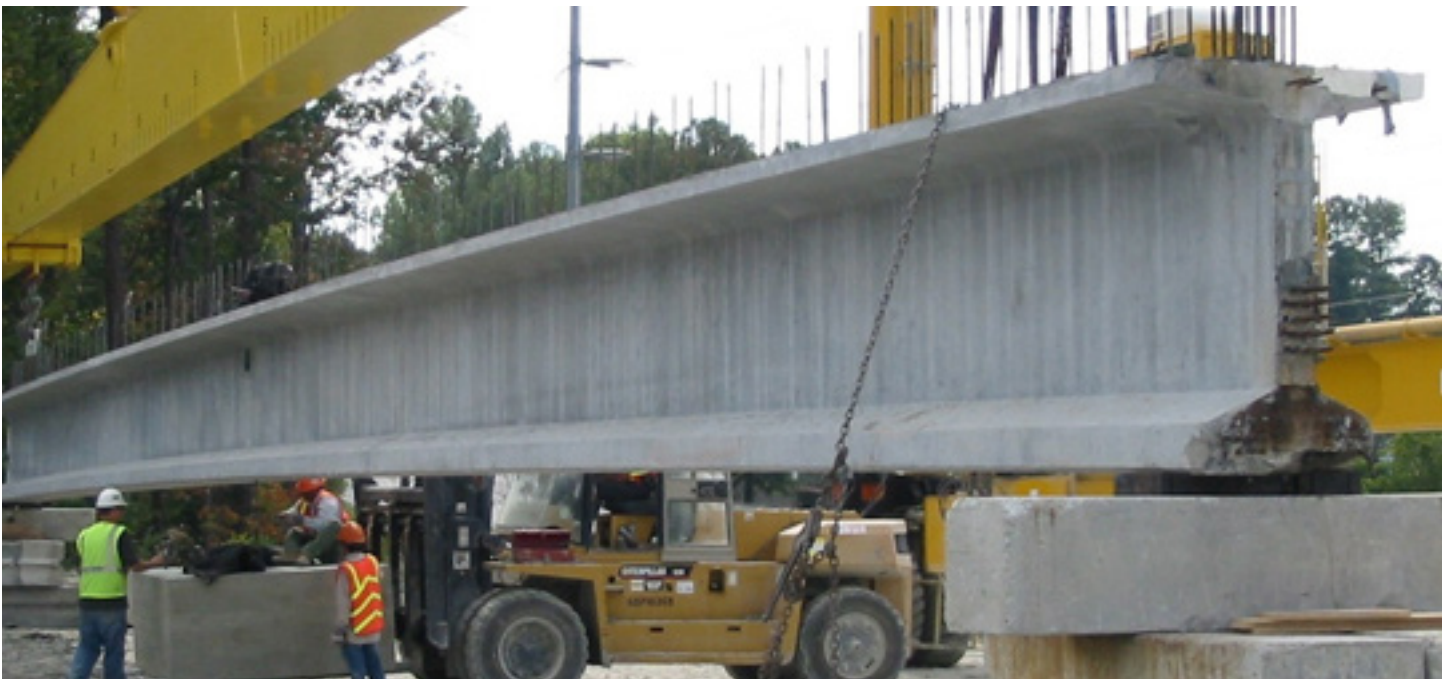
Load test of a high strength lightweight concrete girder
