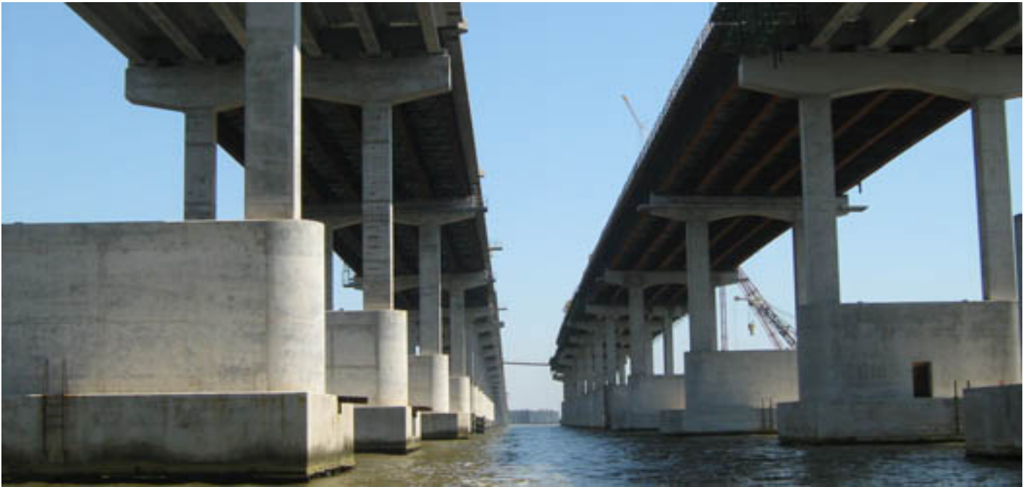
The new bridges were constructed entirely of high performance concrete.
