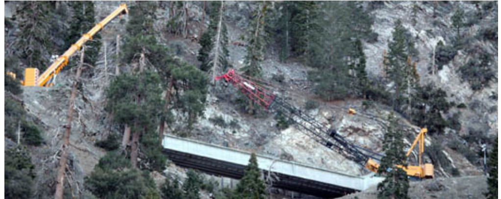
Three different high performance concretes were used in the bridge.
