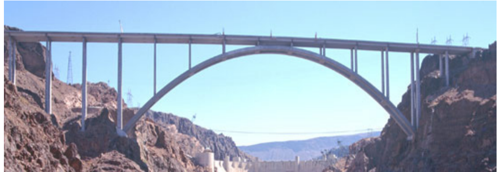
Concrete with a specified compressive strength of 10,000 psi (69 MPa) was used in the arch. Photo: Central Federal Lands Highway Division, Federal Highway Administration
