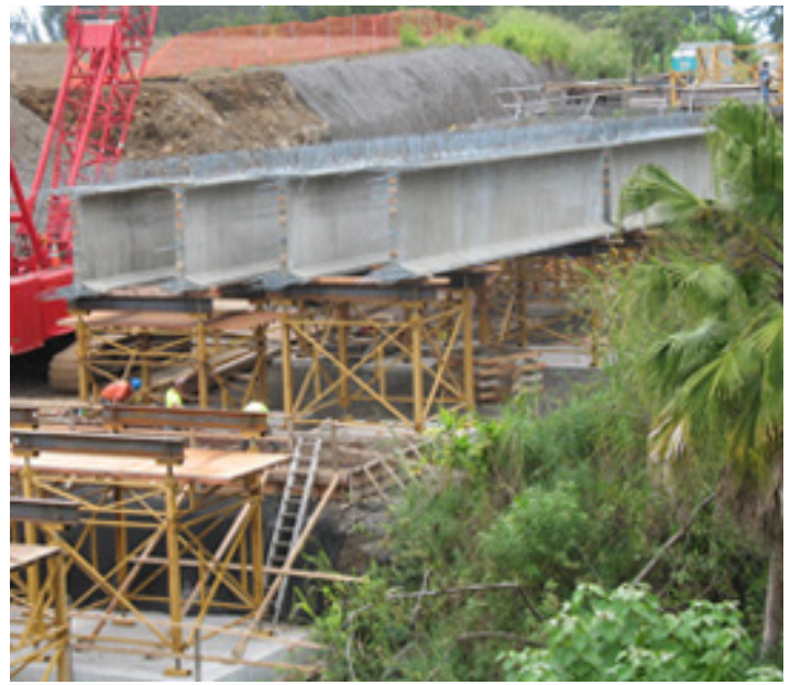
Concrete with a specified compressive strength of 9000 psi (62 MPa) was used in the spliced girders.
