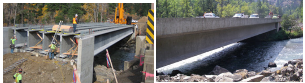
Tieton River Bridge.
