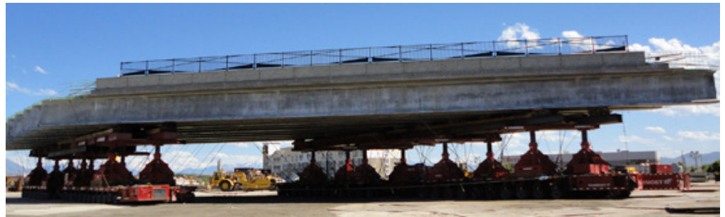
I-15 Prefabricated Bridge Superstructure – Pioneer Crossing, Utah.
