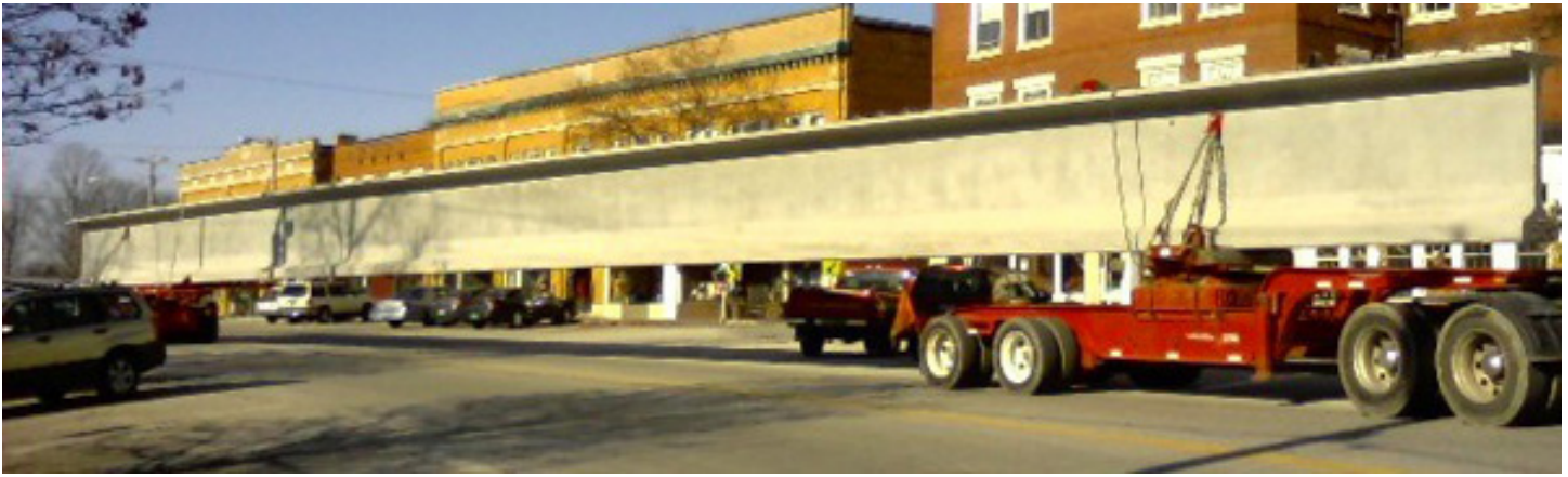
10,000 psi (69 MPa) concrete was used in the beams.
