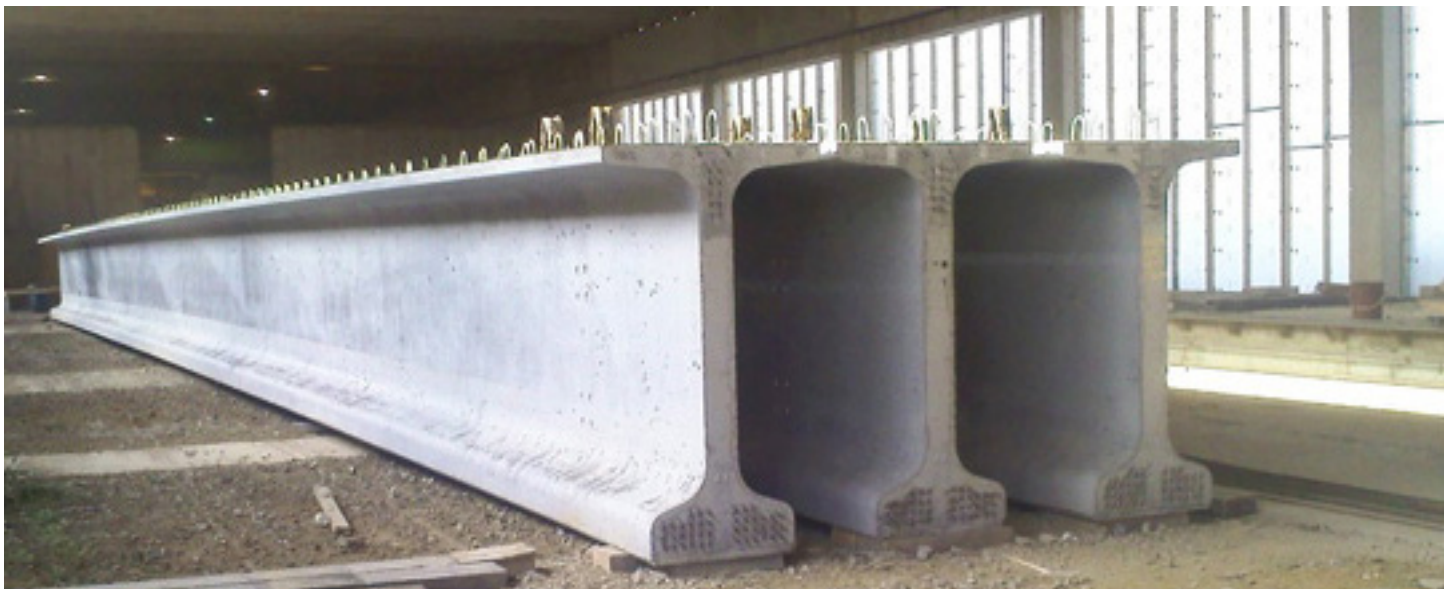
Beams for the Hoosick River Bridge.
