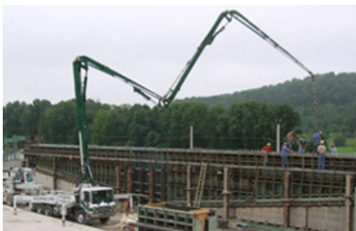
Concrete being placed in the pier segments
