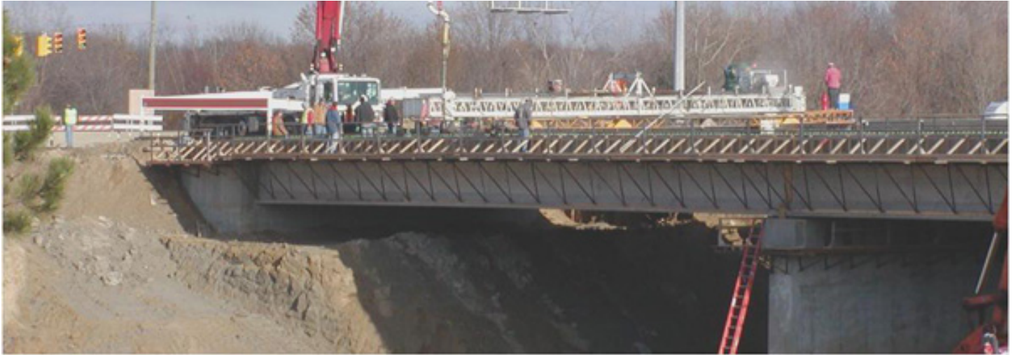
SR 23 bridge under construction using a ternary concrete mix.
