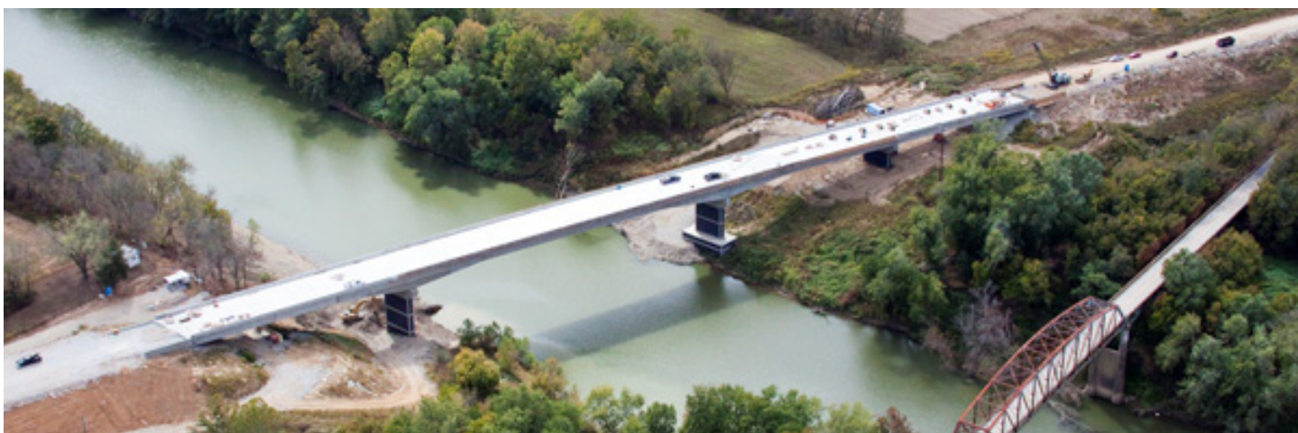
High strength concrete was used for the precast, prestressed concrete beams. Photo: Aerial Innovations of Tennessee, Inc.
