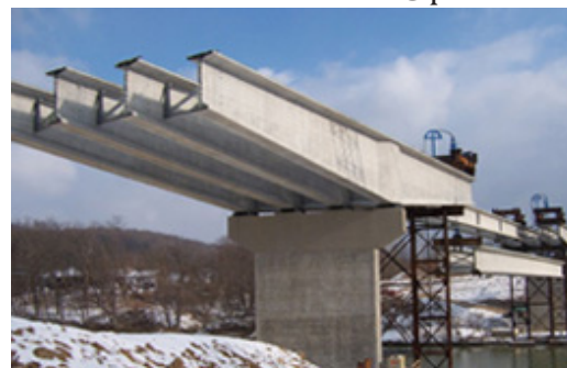
Erected pier segments.
