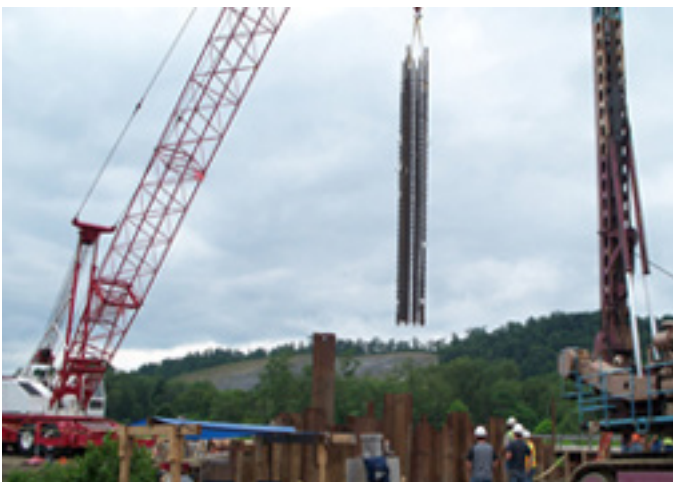
Reinforcement cage being lowered into place.
