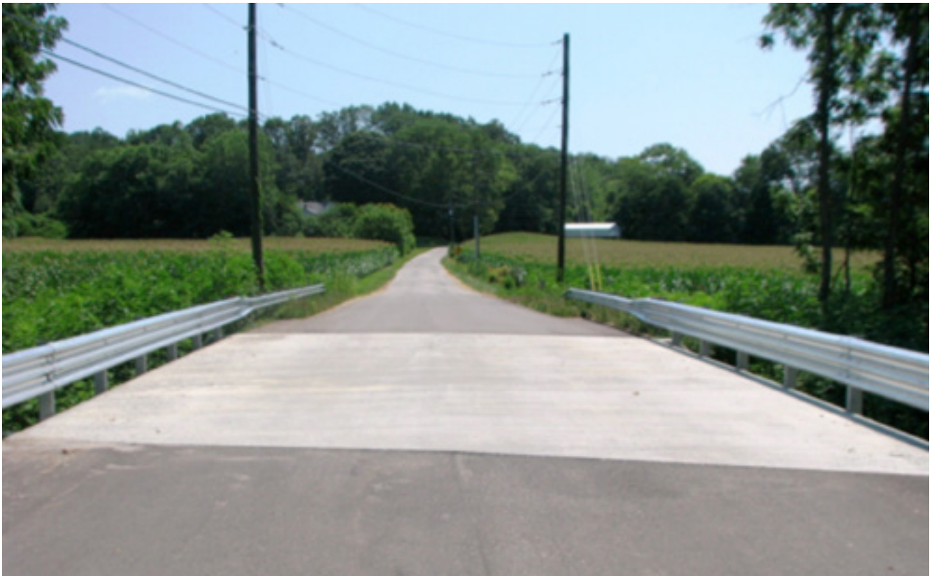
Fig. 3. Currently "crack free" internally-cured concrete bridge deck in Monroe County, Indiana after 1 year in service.
