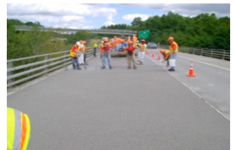
Fig. 4. Inspecting a Bridge.
