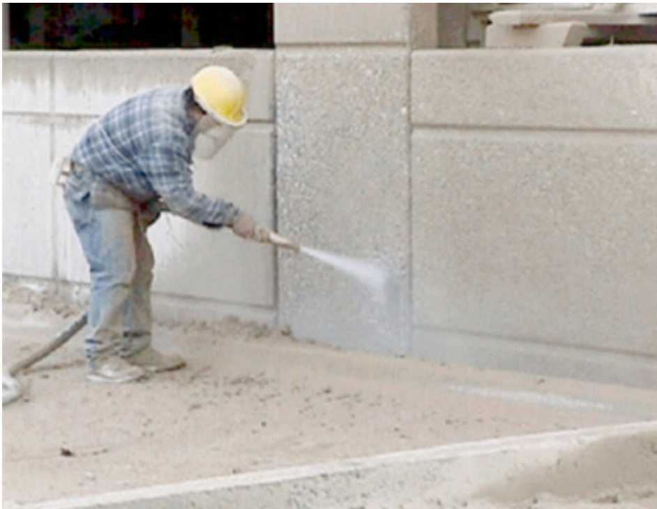
A worker sandblasts a concrete surface.
