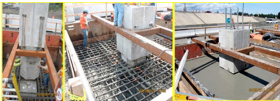
Figure 2: Construction sequences for placement of precast column segment into footing.
