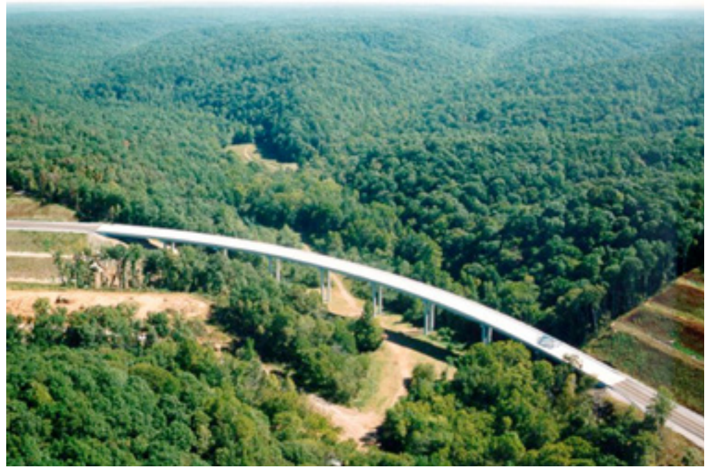
SR-50 over Happy Hollow Creek: Tennessee's Longest Jointless Concrete Bridge at 1175' Long
