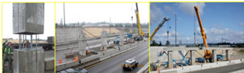
Figure 3: Column Segment and Precast Bent Cap Erection.
