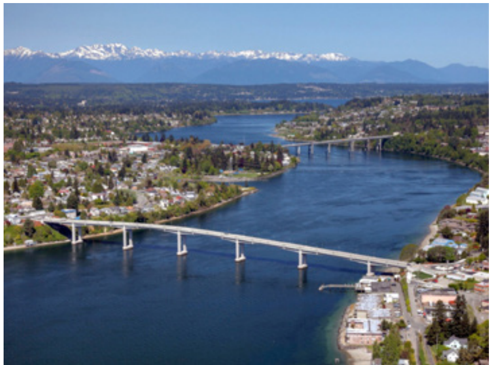
The Manette Bridge in Bremerton, Washington.
