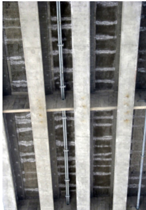
Fig. 2. (left) – View of the underside of a bridge deck constructed in 2010 with conventional bridge deck concrete. Fig. 3. (right) – View of the underside of a bridge deck constructed in 2013 using WSDOT performance-based bridge deck specifications
