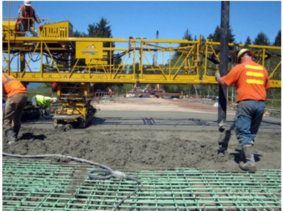
Fig. 1. Bridge deck placement and curing
