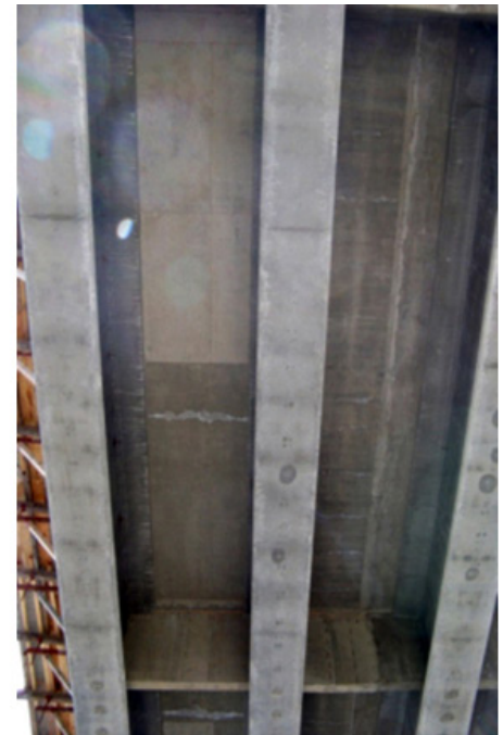
Fig. 2. (left) – View of the underside of a bridge deck constructed in 2010 with conventional bridge deck concrete. Fig. 3. (right) – View of the underside of a bridge deck constructed in 2013 using WSDOT performance-based bridge deck specifications
