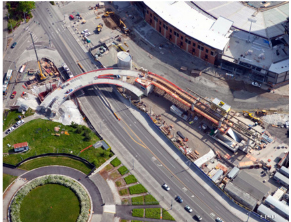
Fig. 1. An aerial photo of the Mountlake Triangle Pedestrian Bridge Project
