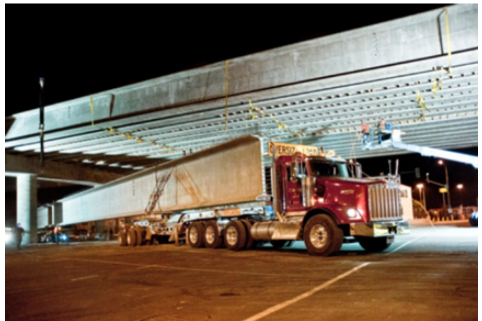
Fig. 1. Owner adopted conservative design policies were used to design 205 ft long precast-prestressed girders in Washington State
