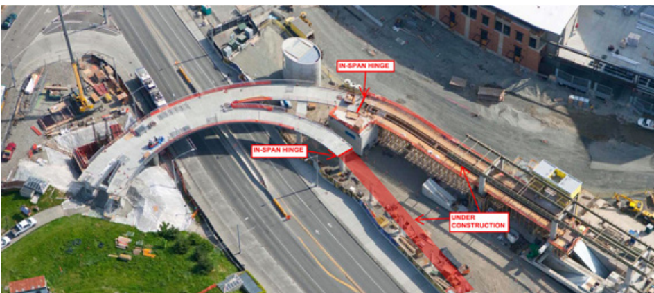
Fig. 2. Identifying the in-span hinges.
