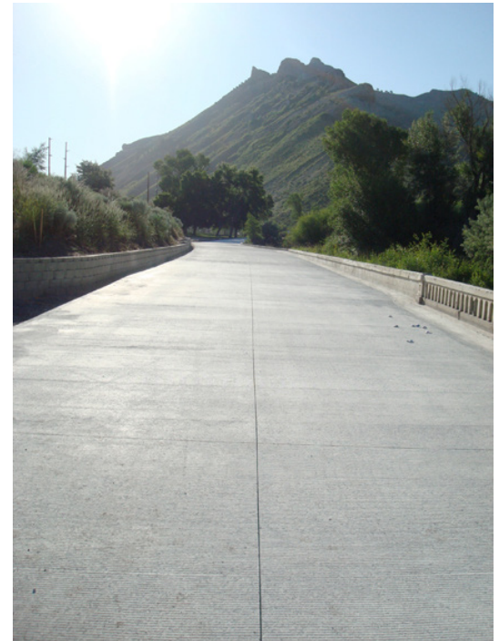
Fig. 1. Lost Creek Road in Morgan UT utilizes PLC cement, and is a major transportation route handling heavy truck traffic for a cement plant
