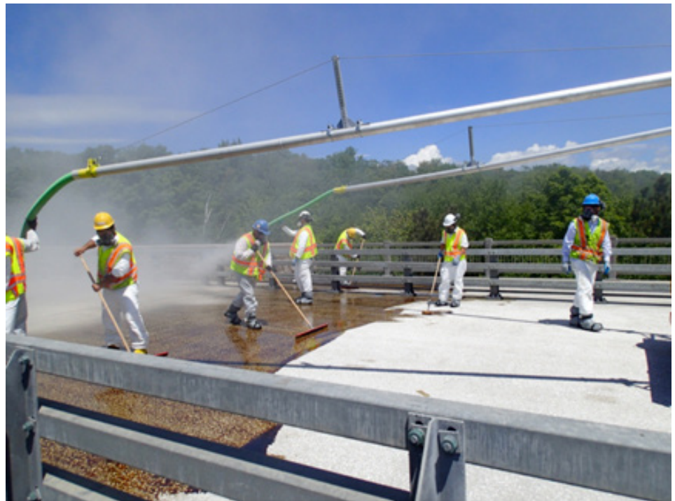
Fig. 1. Michigan Workers Placing Thin Epoxy Overlay on US-2 over the Cut River.
