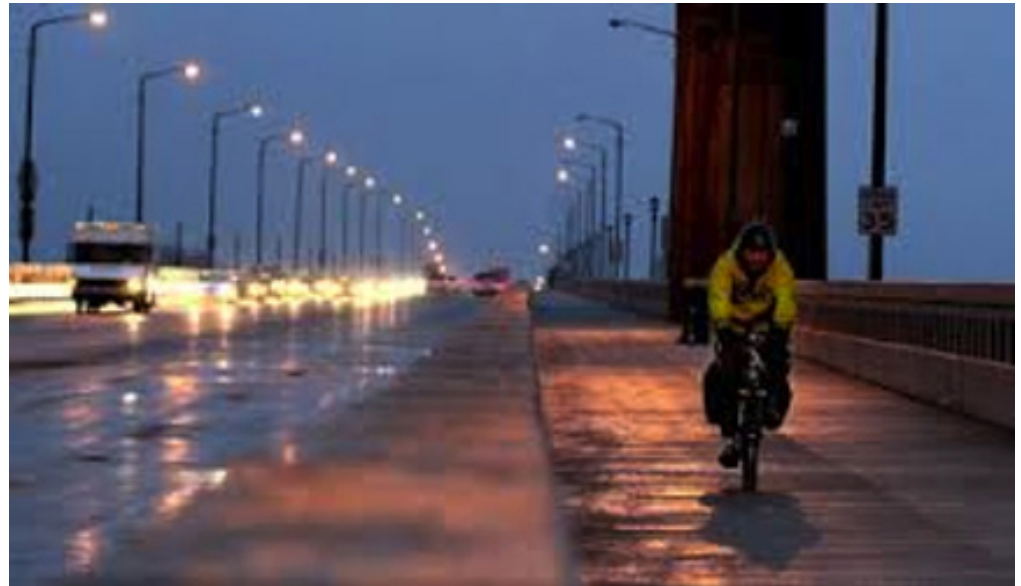
Fig. 1. Nearly 80 years after it was first constructed, the Hope Memorial (Lorain-Carnegie) Bridge is “complete.” In 2013, a protected bikeway opened, making the street safer, more family friendly and conveniently accessible for pedestrians and bicyclists who would prefer not to ride in the street to cross the Cuyahoga River valley. The $4.5 million investment is consistent with the Cleveland’s Complete and Green Streets law, which requires sustainable transportation options be incorporated into new road projects.
