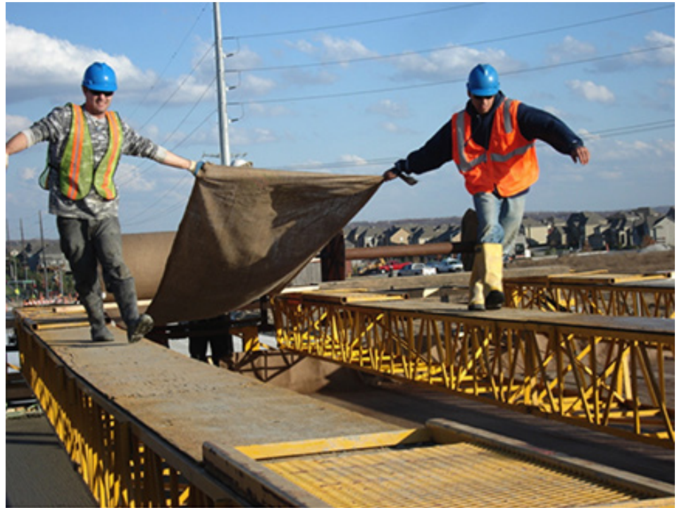
Fig. 1. Pre-cut, rolled, wet burlap is placed within 10 minutes of strike-off.
